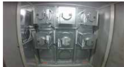
B. After- AHU with redundant and efficient ECFanGrid
