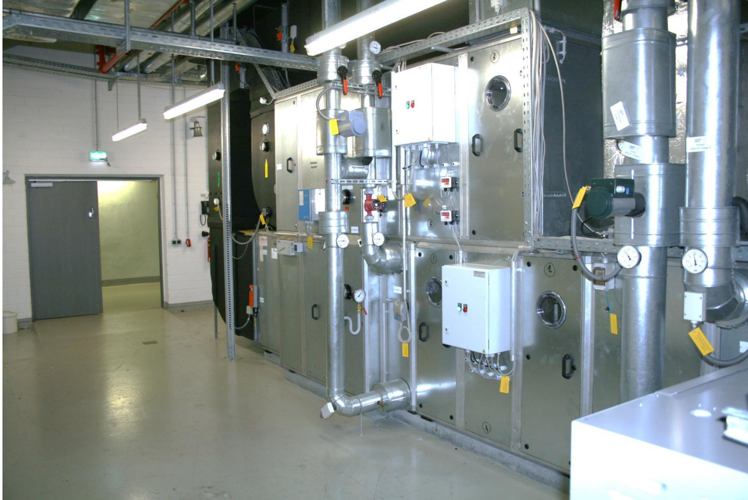
Left. ECFanGrid Retrofit Unit after the installation with wiring cabinets.
